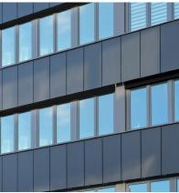
50-year-old building was completely renovated, technically and energetically brought up to date according to Energy Efficiency 100. 234 anthracite-colored SKALA modules were integrated into the facade below the window strips and on the parapets.
