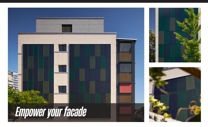
The building envelope of the residential complex was totally refurbished with penthouse apartments. The property rated with an energy efficiency label AA+ generates electricity and hot water via PV modules on the roof, on balcony parapets as well as two SKALA solar facades.
