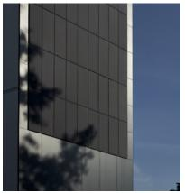
During the renovation of the Stadtwerke Bad Hersfeld high-rise building, the south-east side was extended with a solar facade consisting of anthracite-colored SKALA modules and thus upgraded to an energy-efficient facade.
