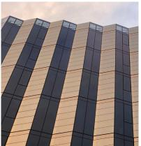
On Australia's first solar facade, transparent window surfaces were combined with opaque solar modules consisting of light grey SKALA modules. The different facade materials are optimally orientated the solar radiation.
